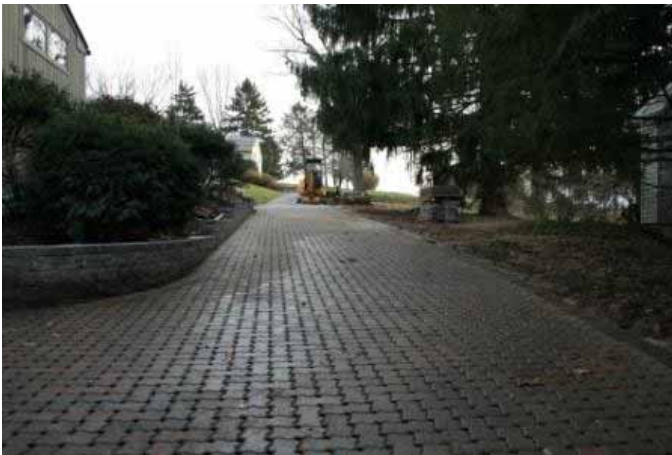
Figure 12. Unilock paver driveway in Middletown, CT. The space between the pavers allows water to infiltrate to a stone base that allows the storage and infiltration of water.
