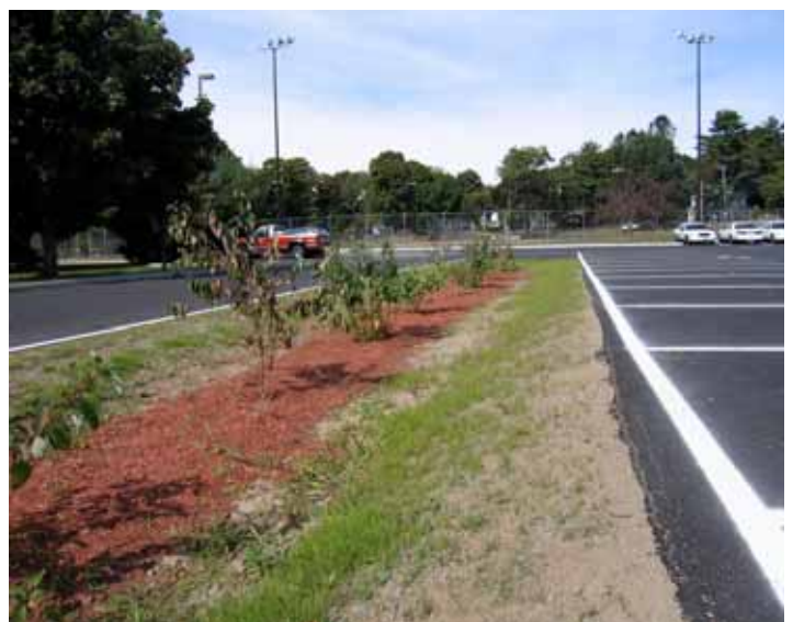
Figure 9. A bioretention area at the Waterford Town Hall parking lot. Simple landscaping practices such as these can treat parking lot runoff while reducing stormwater volume leaving the site.
