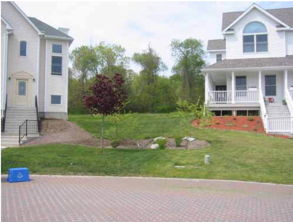
Figure 14. Use of a rain garden, or bioretention basin, to accept roof runoff from two homes in the Glen Brook Green subdivision in Waterford. Other techniques include the use of rain barrels and cisterns for water storage and use for landscape watering.
