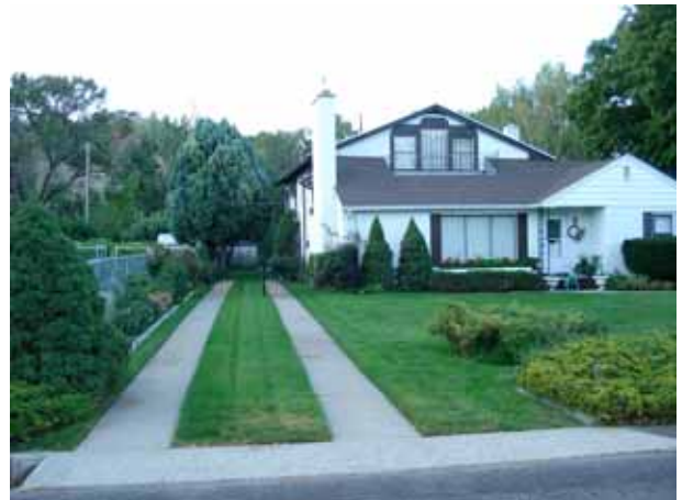
Figure 13. A two track driveway design, once common in early residential development, reduces the total imperviousness of the drive, while preserving the function.
