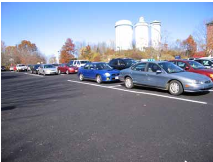
Figure 8. A porous asphalt parking lot at the University of Connecticut. This 106 car lot significantly reduces runoff that would come off a traditional asphalt lot.
