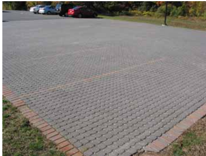
Figure 7. Overflow lot at L&M Hospital out-patient facility in Old Saybrook.
