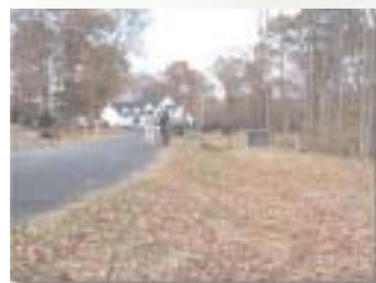
(photo 2) Old Saybrook model stormwater subdivision, showing grassed swale drainage system.
