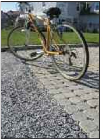
Public access parking stalls at Cornfield Point, Old Saybrook feature pervious pavement. Shown here are both modular concrete pavers and Gravel Pave2™.
