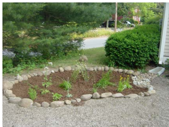
Roof runoff should be directed to pervious vegetated areas, such as this rain garden.
