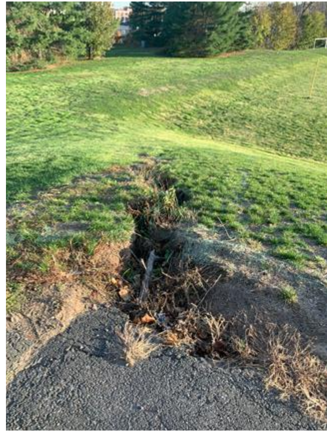
Erosion at the corner of the building
