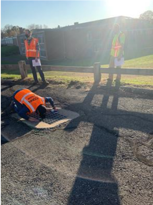
Catch basin - overloaded by runoff from the parking lot
