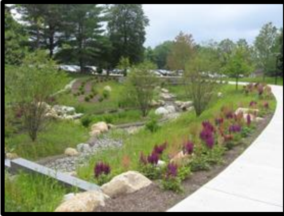
Rain Gardens and Bioretention
