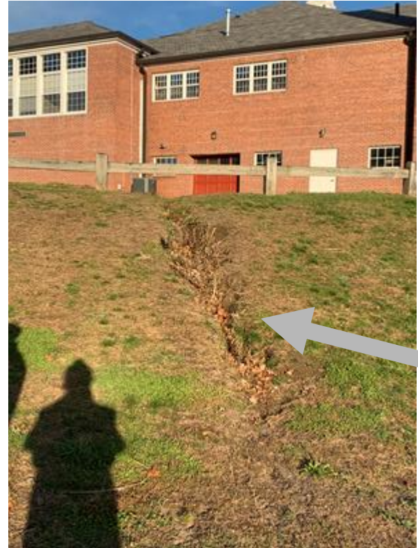
Erosion caused by the overflow in the catch basin
