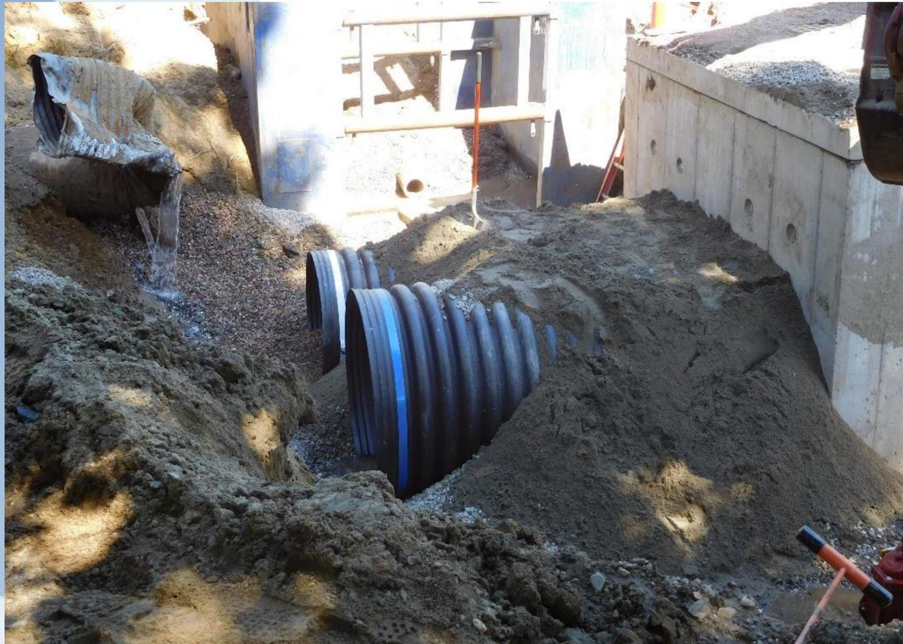
**Dual Pipe Installation - The project replaced old and undersized drainage pipe to prevent flooding and slow the rate at which stormwater flows to Bartlett Brook**
