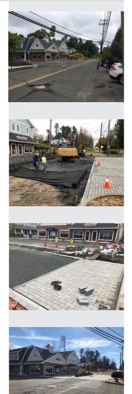
Images of Trumbull's phase one construction and finished pervious pavers
